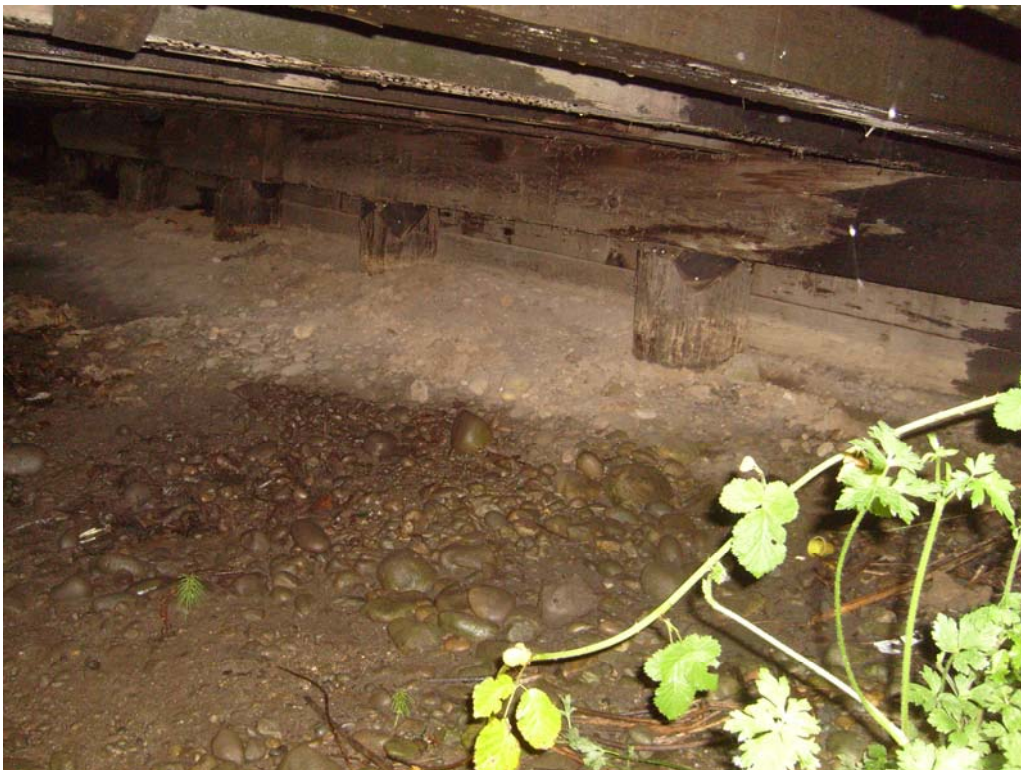
Photo No. 6: Pier 3 looking northwest.
