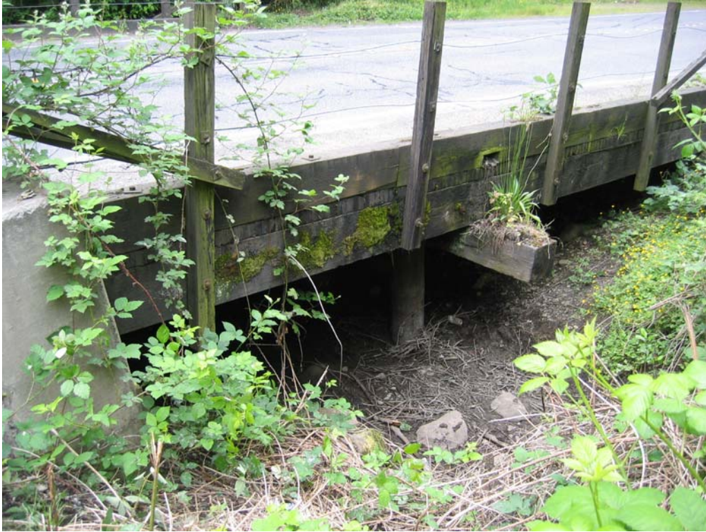
Photo No. 3: Elevation looking west.
