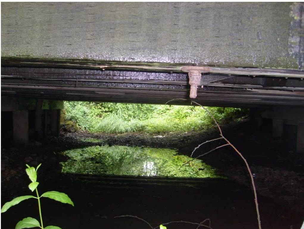
Photo No. 4: Elevation looking west.
