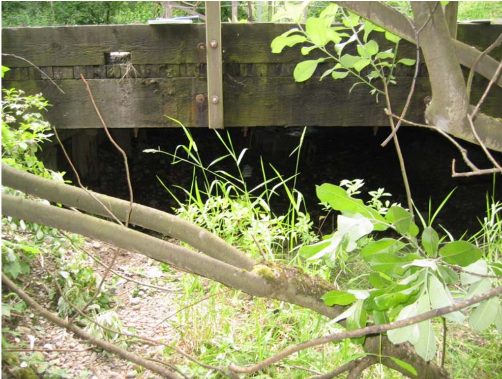
Photo No. 3: Elevation looking west.
