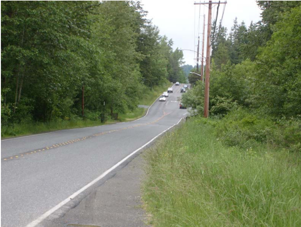
Photo No. 1: Roadway Deck looking north.
