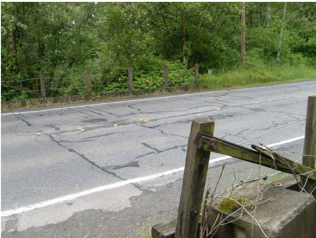
Photo No. 2: Roadway Deck looking northwest.
