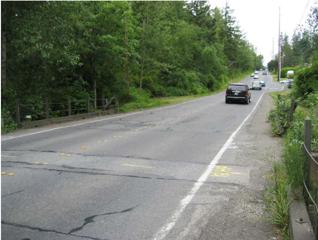
Photo No. 1: Roadway Deck looking north.
