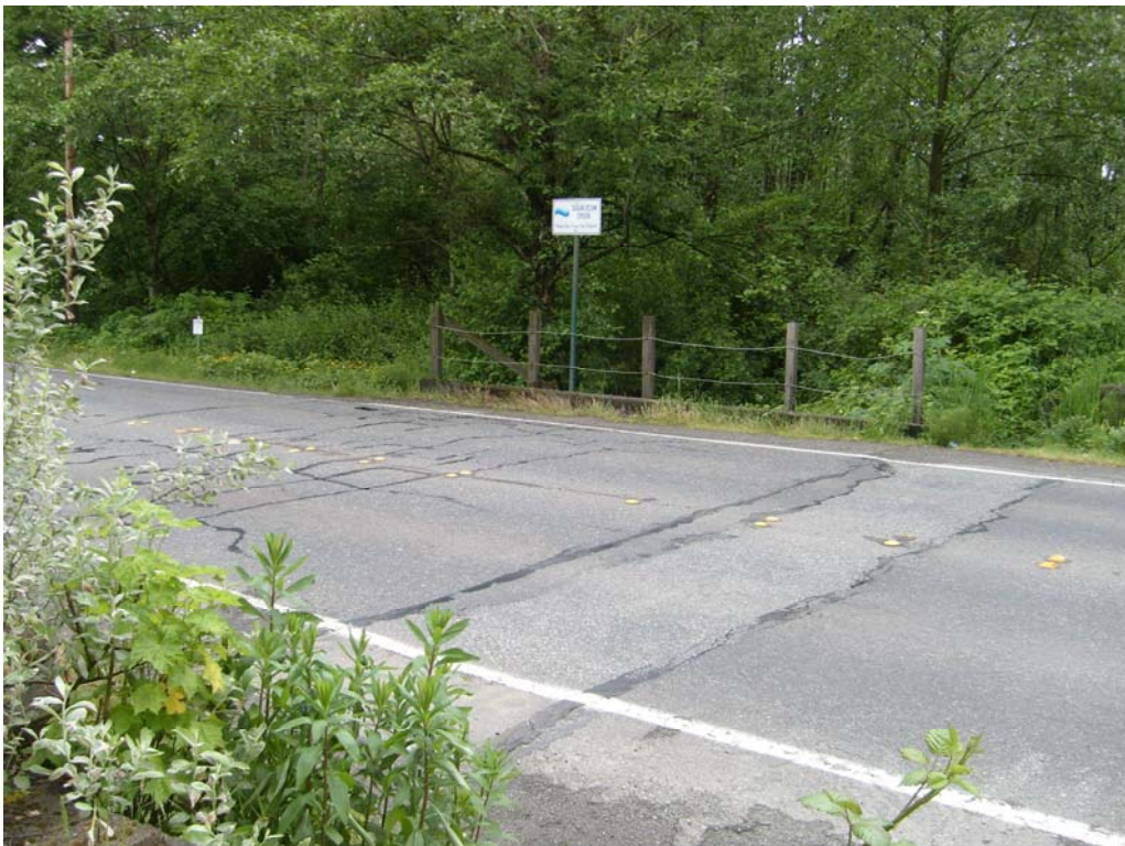
Photo No. 2: Roadway Deck looking southwest.
