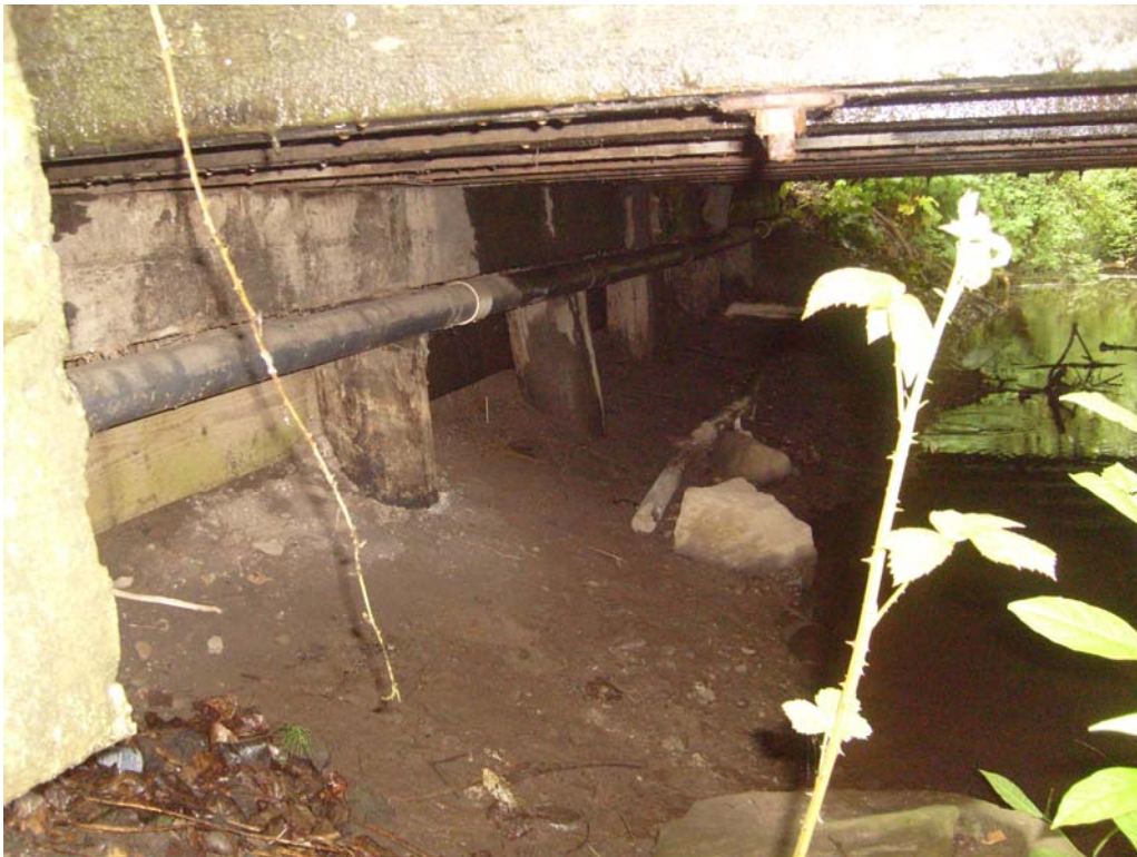
Photo No. 4: Pier 1 looking southwest.
