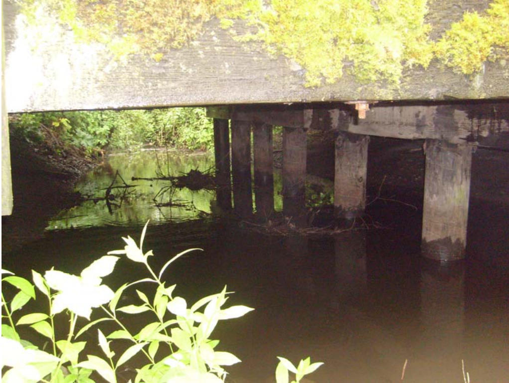
Photo No. 5: Pier 2 looking northwest.
