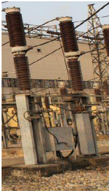
Figure 5.11: Minimum oil CB.
