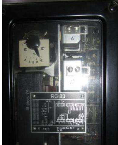
Figure 4.4: Negative phase sequence relay.
