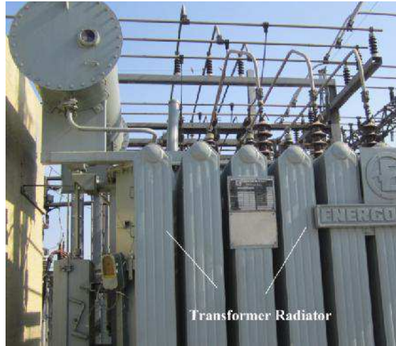
Figure 4.16: Transformer radiator for oil filled safe cooling.
