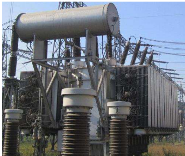
Figure 5.9: Intermediate potential transformer.
