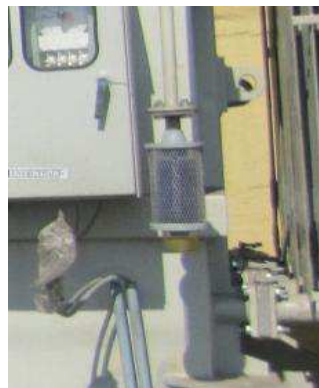
Figure 5.4: Breather of a power transformer.
