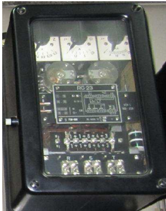
Figure 4.6: Generator Differential Relay.
