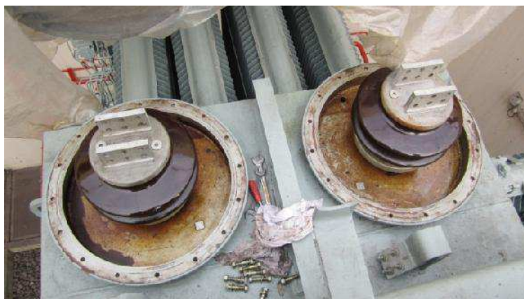
Figure 5.25: Primary bushing of a single phase unit transformer.
