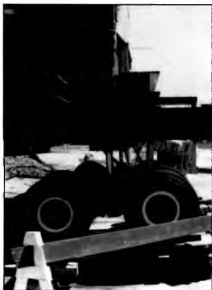
March 1991 photo of "moving day" with the front part of the house raised onto steel "pins" (small lateral, closely placed beams) which in turn rest on large transfer beams supported by hydraulically-leveled dollies. The back pre-1913 wing has been carefully dismantled and stored for future re-erection (Peril Two).
