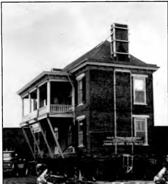
March 1991 photo of "moving day" with the front part of the house raised onto steel "pins" (small lateral, closely placed beams) which in turn rest on large transfer beams supported by hydraulically-leveled dollies. The back pre-1913 wing has been carefully dismantled and stored for future re-erection (Peril Two).
