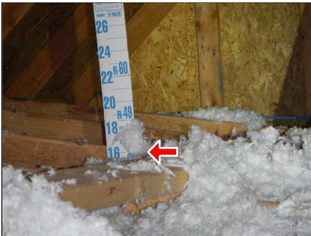
9.2 Picture 1 Good insulation in attic
