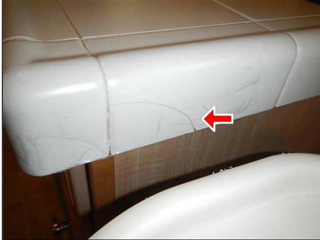
4.5 Picture 1 Small hairline crack in kitchen countertop.
