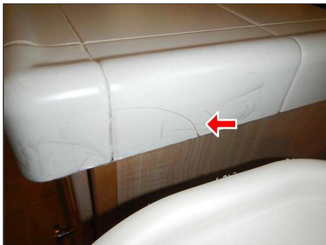
4.5 Picture 1 Small hairline crack in kitchen countertop.
