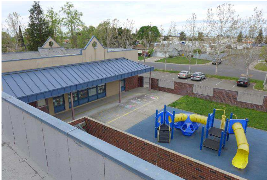
View of the kindergarten play area from Glenwood Elementary roof. (Credit: CFW, Inc.)
