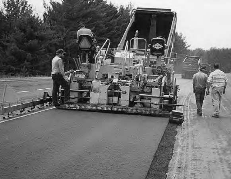
Road construction projects benefit from a bid process that attracts competitive bids from reputable contractors.
