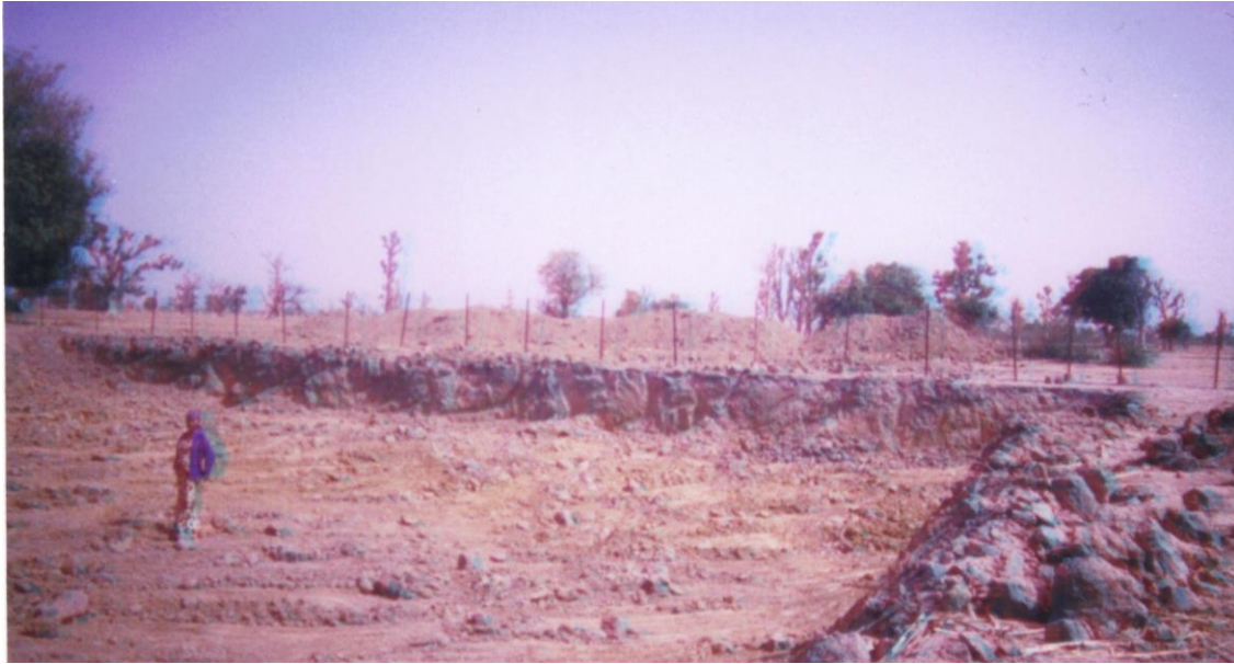
Figure 12 A recently dug catchment by an Engineering Without Borders group
