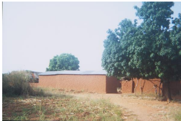
Figure 7 Types of roofs in Mali
