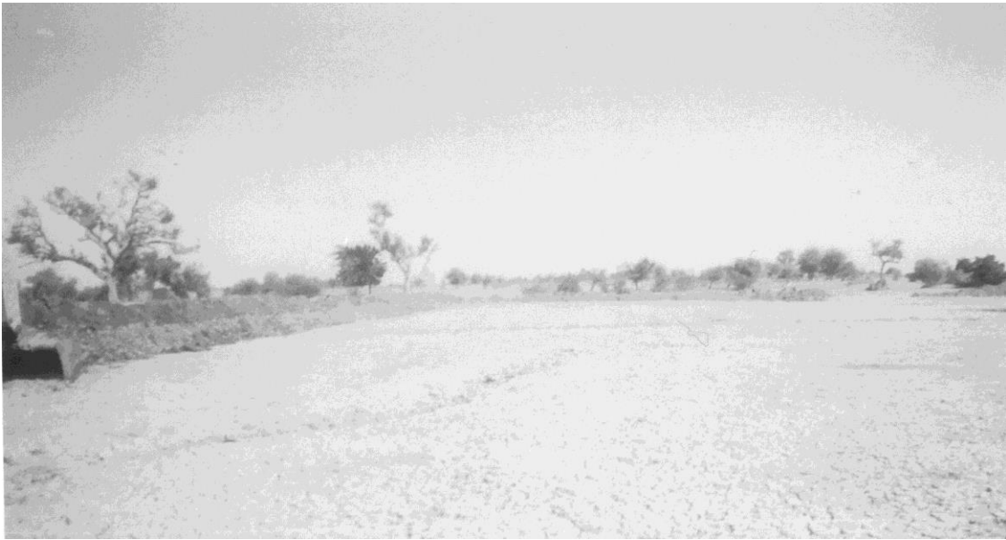
Figure 11 The Kamian Catchment excavation in progress (100m by 80m by 1.5m)
