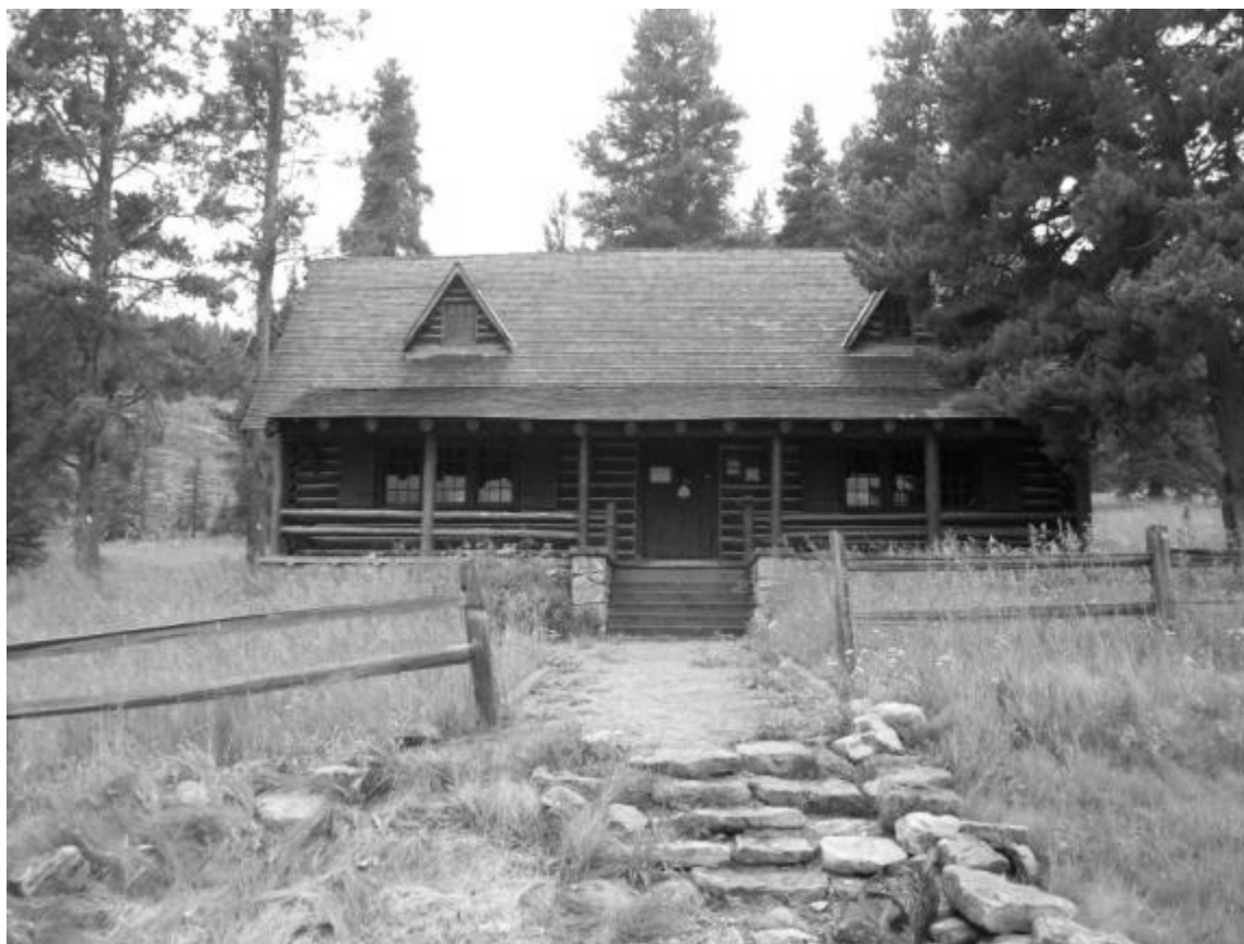
Photo 4. View of the north side of the building.
