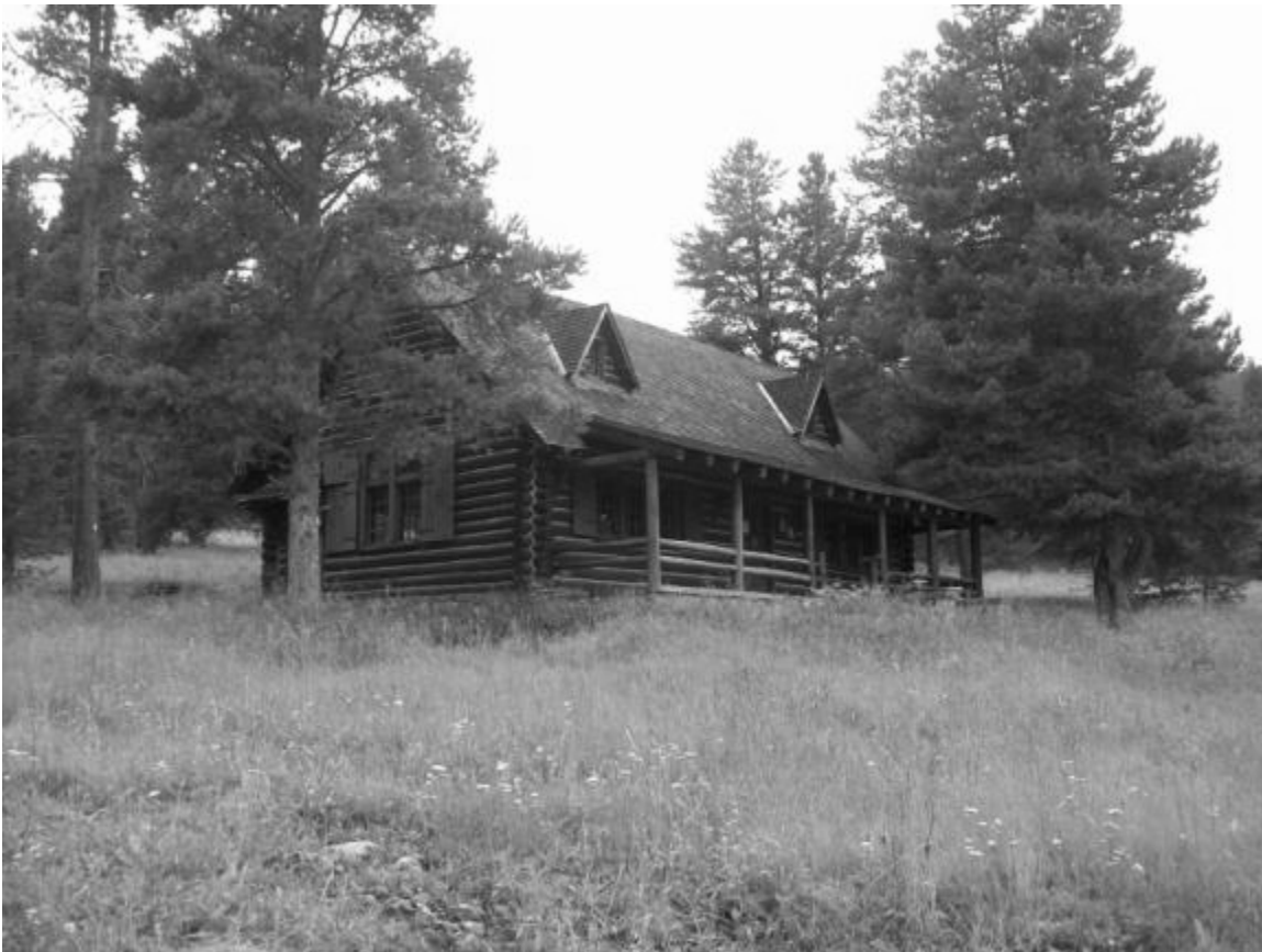
Photo 1. View of the north and east sides of the building.
