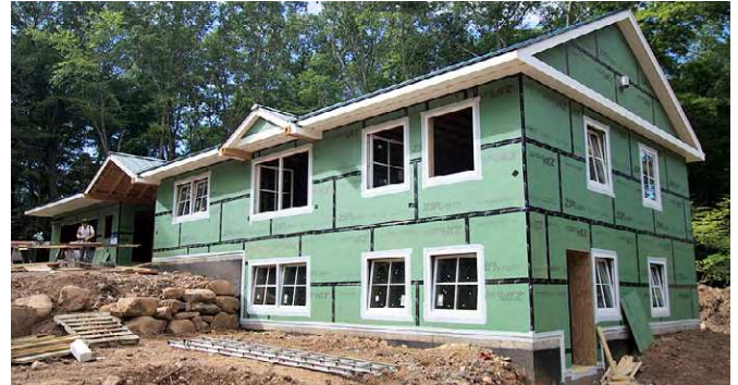
2013 Zero Energy Challenge co-winning home located in Farmington, CT.
