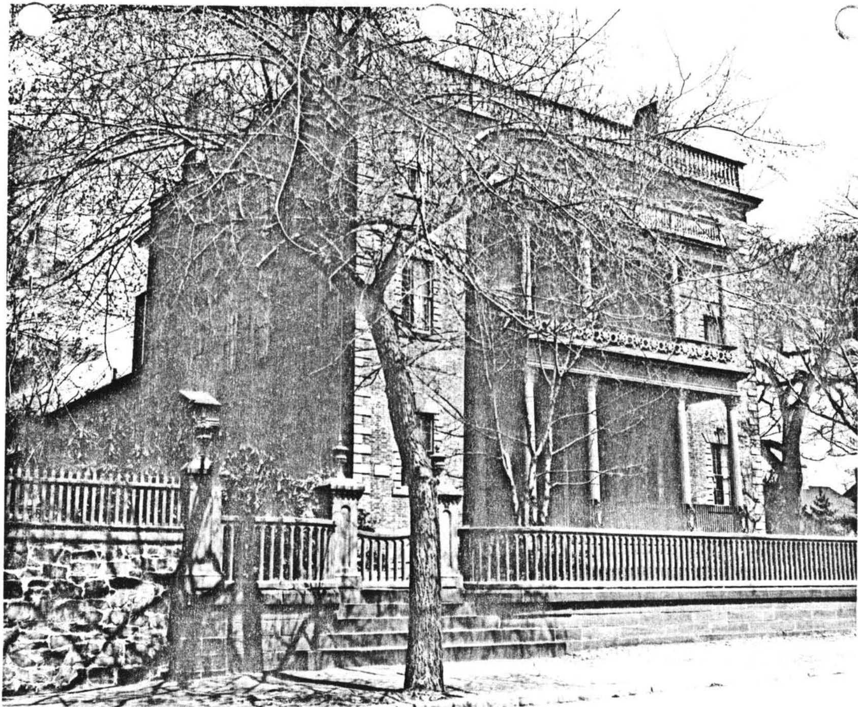
Edward Carrington House, Providence, Rhode Island
