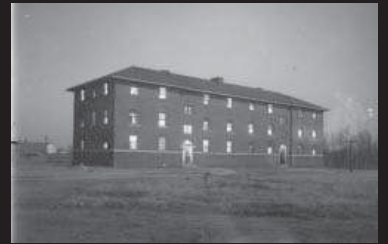
Construction began on the Boys' Dormitory, fifteen years after the University was founded. The original room and board package was $5.00 - $5.50 per month!
