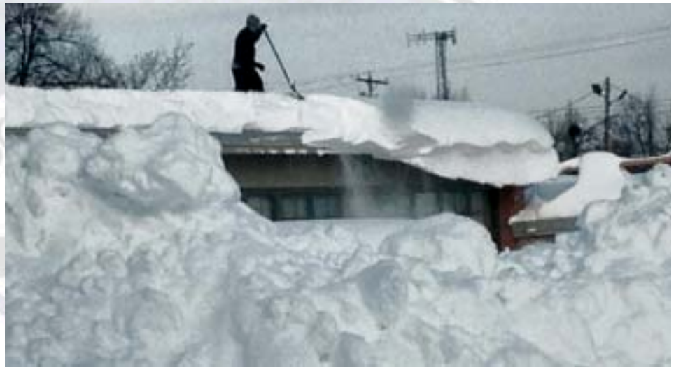
Clearing snow off of the school roof.
