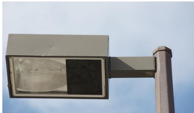
Figure 11: Incumbent 250W HPS roadway luminaire
