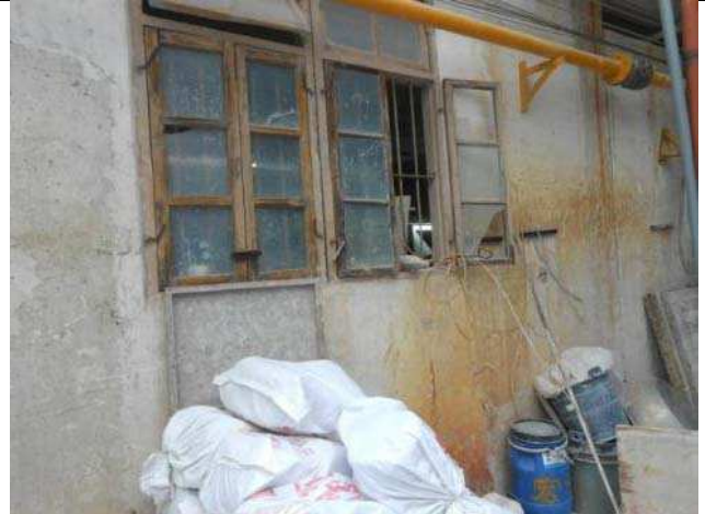
NC 1.3: One piece broken glass was found at WIPs storage area in kiln workshop and four pieces of broken glasses were found at clay storage area.
