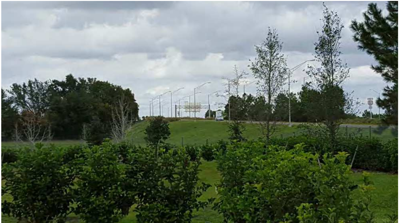
Looking north at Highway 429 Exit Ramp
