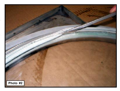
**IMPORTANT**: When working the glass into place, the tendency is there to put force on the glass with the other hand. Be careful not to put too much force on the glass as it will fall through, and you will have to start all over again
