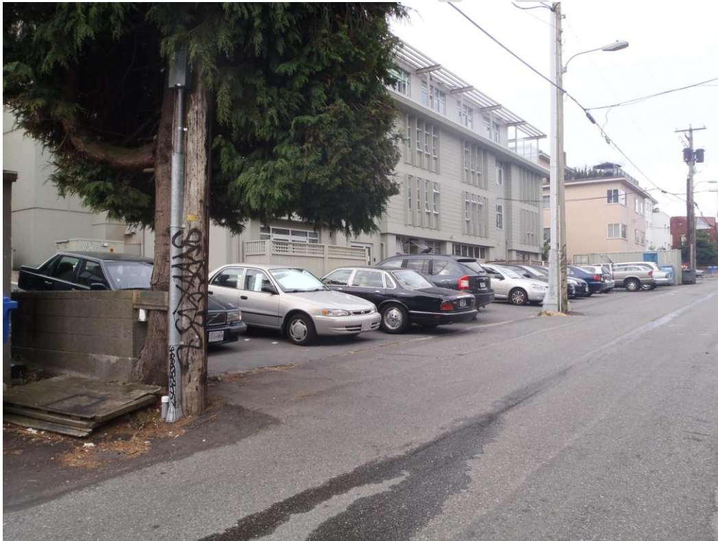
Figure 6 – On-Site Parking along Backlane
