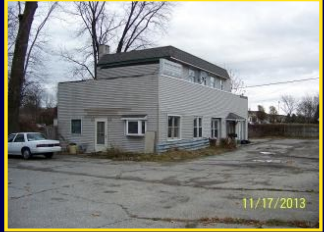
WEST SIDE OF PROPERTY & FRONT PARKING
