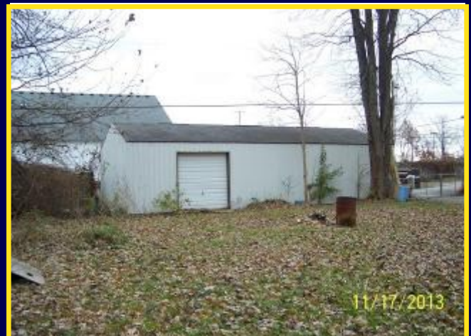
GARAGE ON EAST SIDE OF PROPERTY
