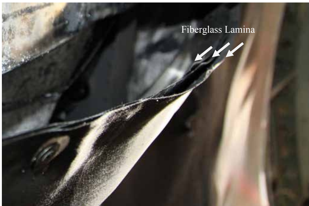
Figure 25. Cargo Liner Delamination
