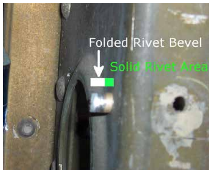
Figure 34. Rivet With Bracket Pulled off Beveled End
