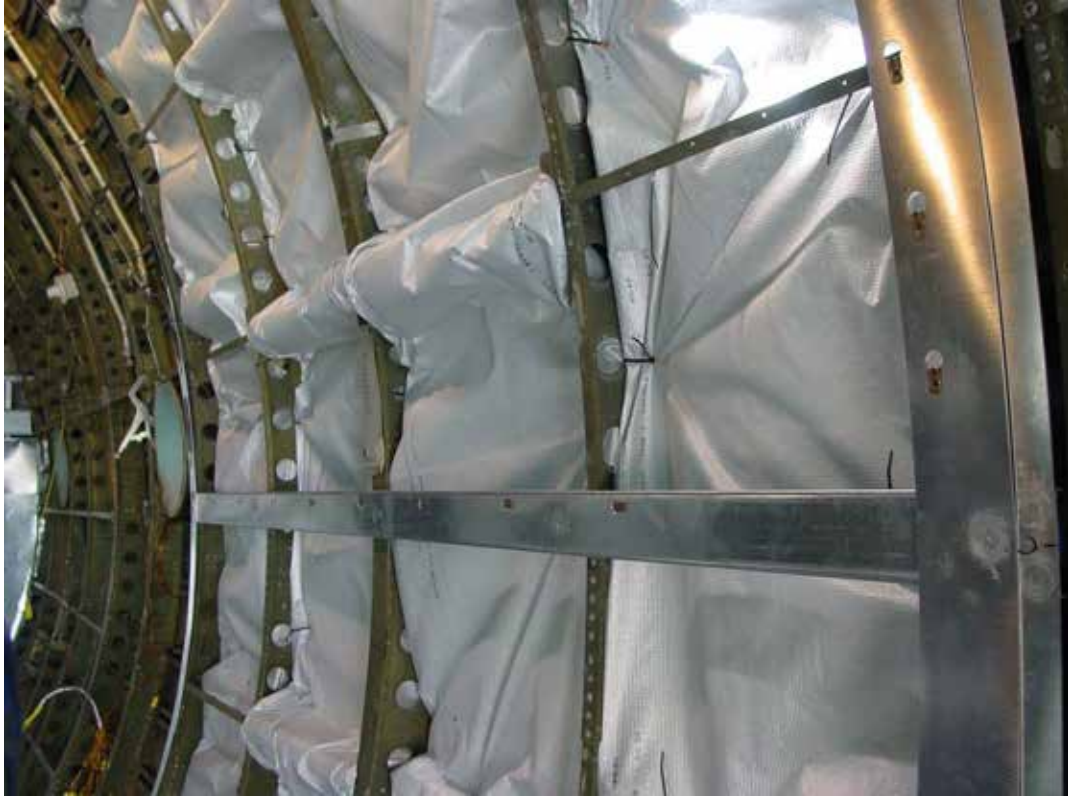
Figure 13. Test Section With Insulation Blankets and Framing Installed
