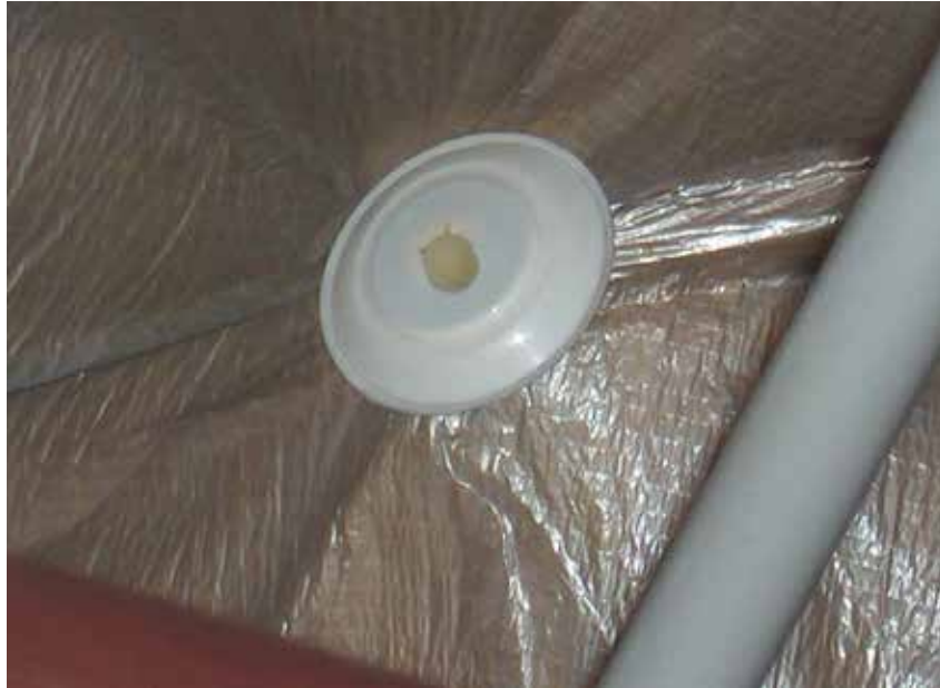
Figure 3. Plastic Insulation Retention Pin and Clip
