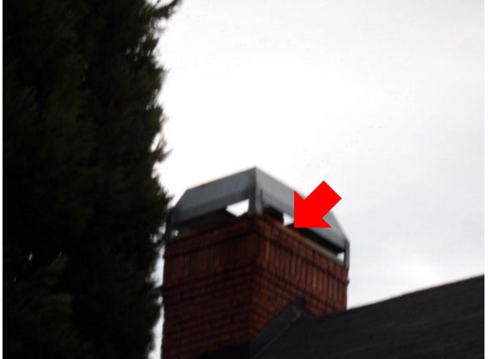
The chimney cap is rusting. Recommend sanding and painting cap.
