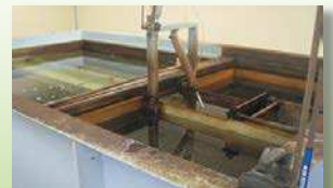
Drinking Water Treatment Plant
