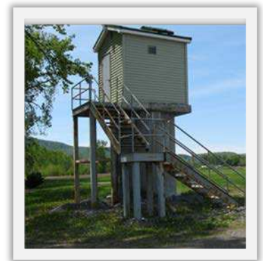
Wellhead above 100-year flood
