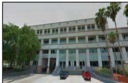
Grizzle Building 2 nd Floor Interior Renovations, Largo Florida Department of Management Services
