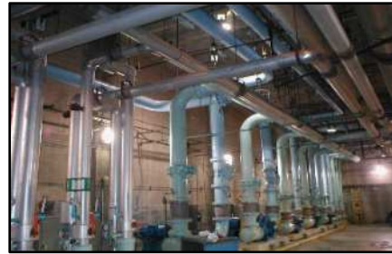
Tampa Convention Center HVAC Improvements City of Tampa
