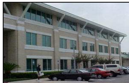
Jacksonville Regional Service Center - Interior Renovations
