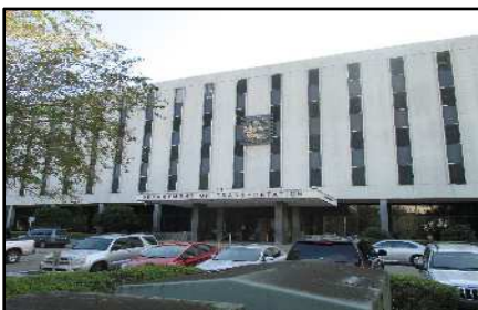
Burns Office Building 2011 Renovations Florida Department of Transportation
