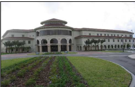
Campus Administration and Instructional Facility University of South Florida, Sarasota / Manatee Campus
