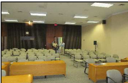
Burns Building Auditorium Renovations 2014 Florida Department of Transportation
