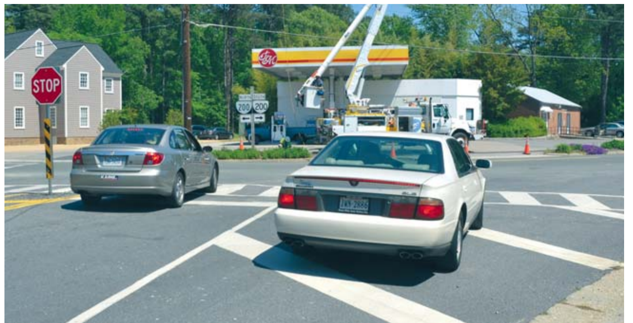
Irvington officials hope to make the intersection above safer by creating a right turn "slip lane" where King Carter Drive meets Irvington Road. Although the street appears wide enough to accommodate two vehicles at the intersection, the white car attempting a right turn above should be in the designated lane to the left—until the Virginia Department of Transportation changes the road markings. Photo by Lisa Hinton-Valdrighi
