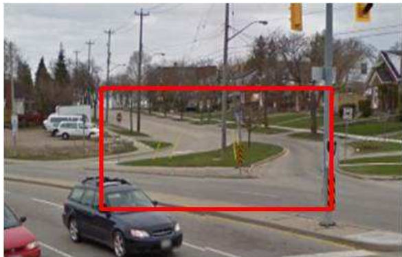
Figure 13 – Intersection Channelization and Right-in/Right-out Island, Kitchener, ON
