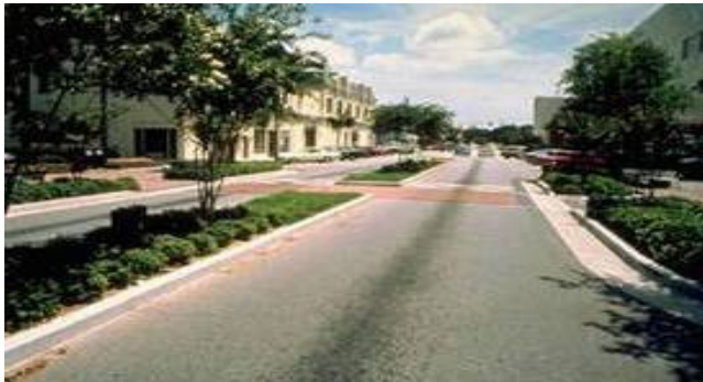
Figure 8 – Raised Median (with Textured Crosswalk) 13
