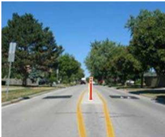
Figure 1 – Speed cushion with Mountable Centre Median, Oakville, ON 8
