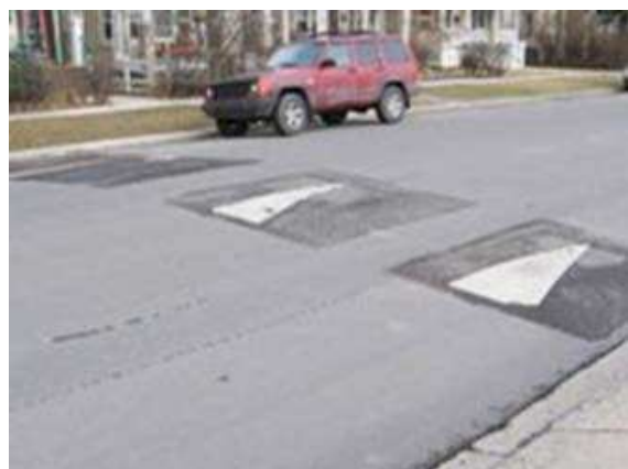
Figure 3 – Speed Cushions for Emergency Vehicles 10
