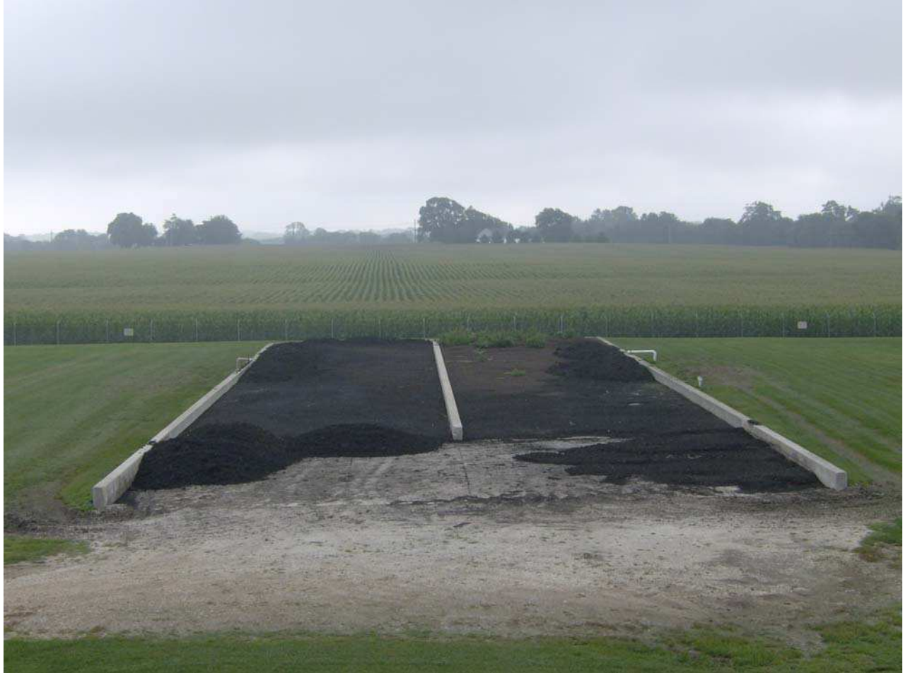
Dewatered Sludge Storage
