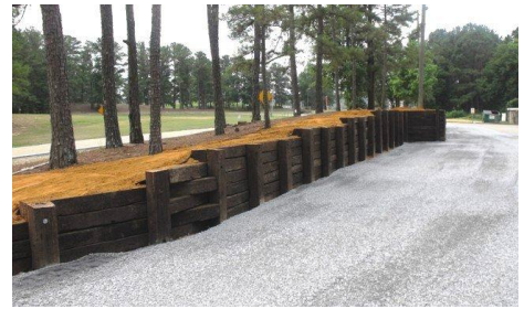
New Retaining Wall & Gravel
