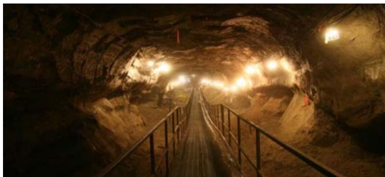
U.S. Army Corps of Engineers A view inside Alaska's unique permafrost research tunnel.
