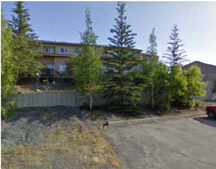
Figure 2 – Rycon Retaining Wall
