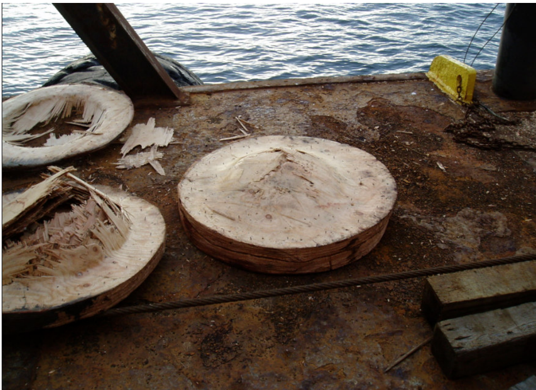
Figure 17: Photograph of one of four previously used 4-inch thick plywood stacked disks that formed the wood pile cap for the concrete piles.
