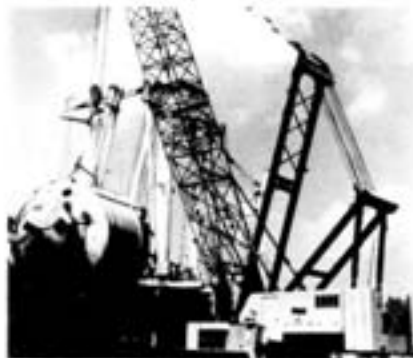
Five 300-Ton Mobile Cranes
