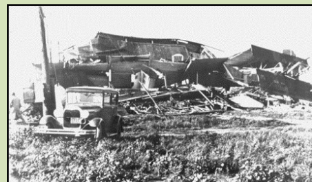
Above: Wood-frame building in Long Beach, CA destroyed by the March 11, 1933, earthquake. Image: USGS
