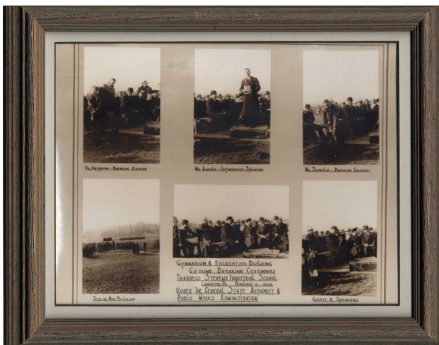
This collage, which shows the groundbreaking ceremonies for the gymnasium and recreation building, is from Tom Beck's photo collection.
