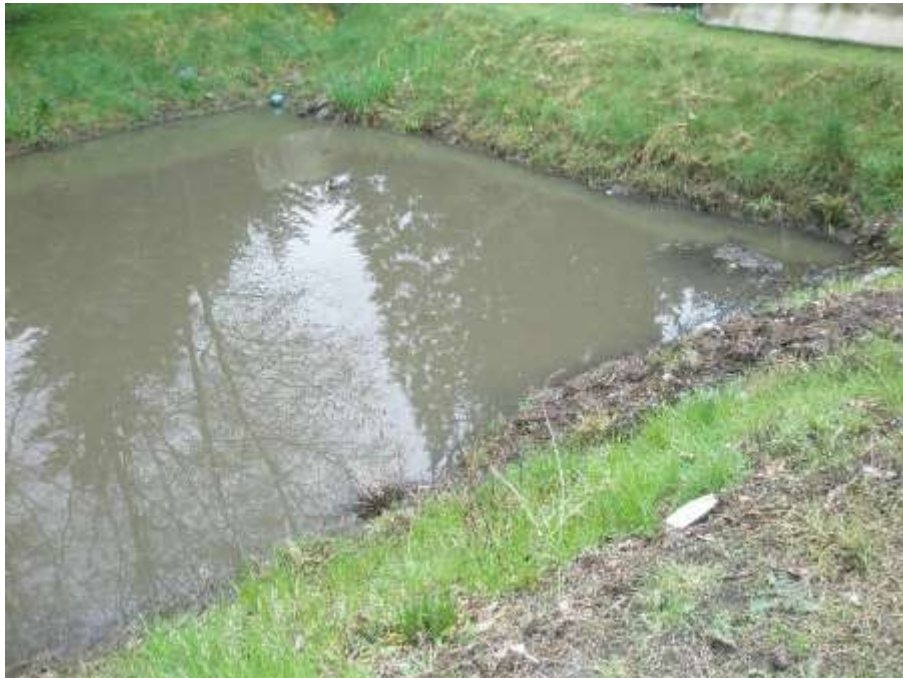
Figure E-8 Stormwater retention pond at Ballinger.
