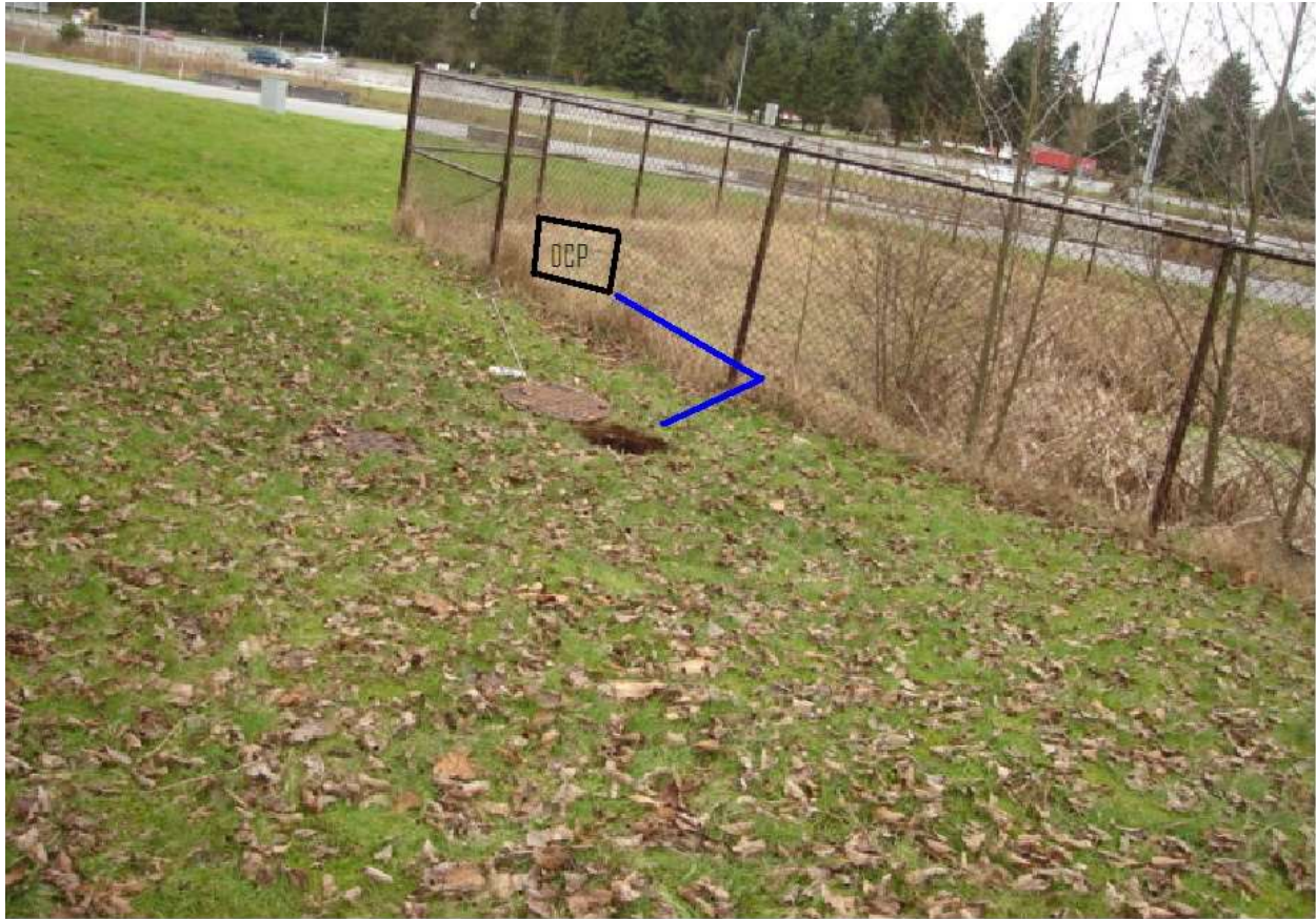
Figure E-12 Location of DCP and monitoring from pipe leaving the oil/water separator at the Smokey Point (NB) Rest Area.
