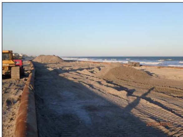
Photo 9. View of the material from the rock boxes being stockpiled seaward of the landward shore pipeline near Sta. 680+00 and 677+00, looking north.
