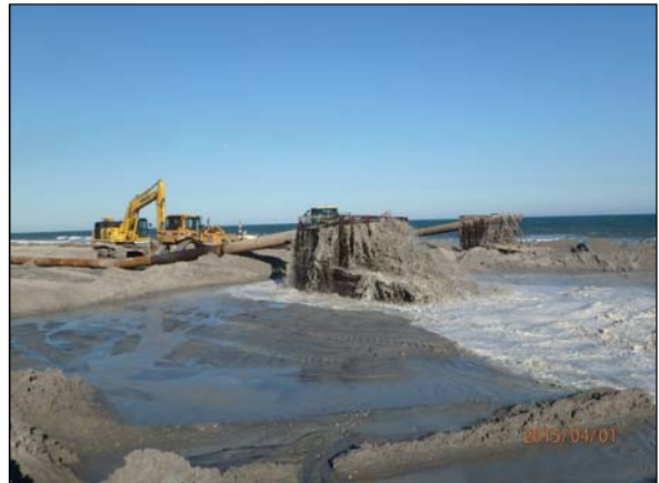
Photo 2. View of the landward and seaward outfalls and rock boxes at 17:45 near Sta. 674+00, looking northeast.
