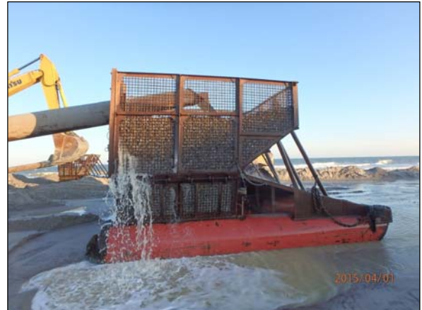
Photo 4. View of the full rock box with the 1.5 inch mesh overlaid on top of the 2 inch mesh.
