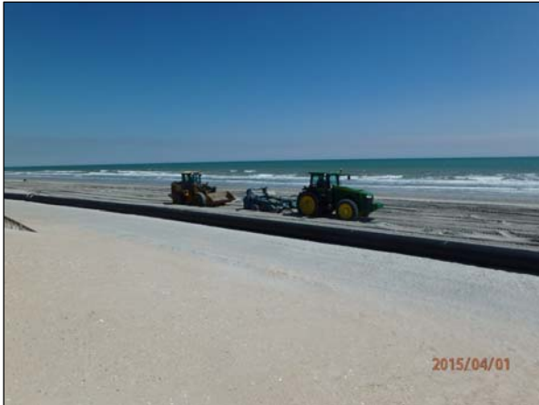
Photo 15. Tigerhole Landscaping commenced rock picking operations up to 36 inches below the constructed grade of the berm area between Sta. 720+00 and 715+00.
