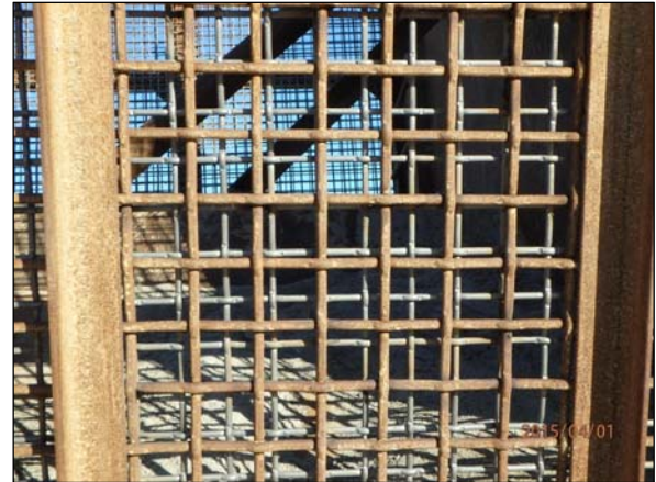
Photo 6. View of the rock box with the 1.5 inch mesh overlaid on top of the 2 inch mesh.
