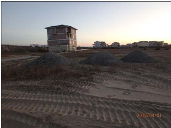
Photo 19. View of the material from Tigerhole Landscaping's rock picking operations being stockpiled at the lot 2 blocks south of the Gray Street access.
