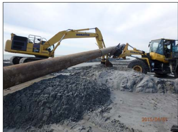
Photo 8. An excavator being used to collect the material from the rock boxes within the discharge area.
