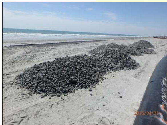
Photo 10. View of the rocks previously collected by the rock picker being stockpiled seaward of the shore pipeline near Sta. 694+00.
