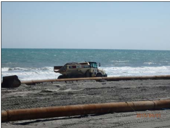
Photo 17. The Town's off-road truck was utilized to relocate 3 truck loads of rock (36 cy) that were removed by Tigerhole Landscaping's rock picker from the constructed berm area between Sta. 720+00 and 715+00.
