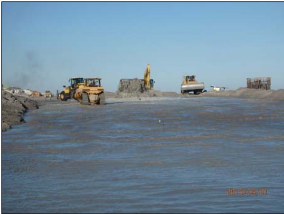
Photo 3. View of the landward discharge area at 17:50 near Sta. 674+00, looking north.
