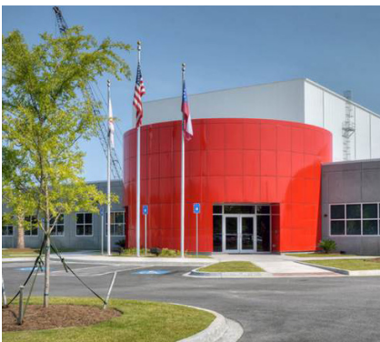
2013 Industrial Award of Excellence in Electrical Construction Winner Mitsubishi Power Systems Americas – Savannah Machinery Works by Excel Electrical Technologies
