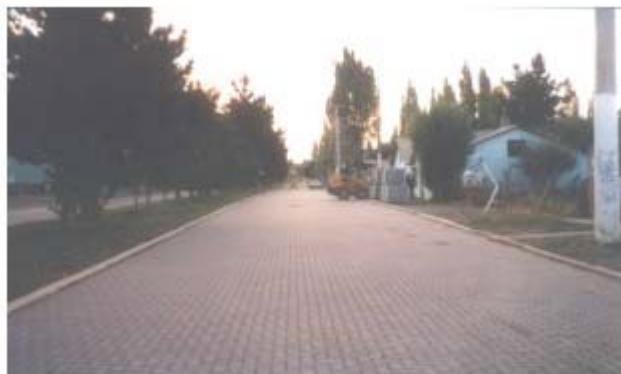
Figure 5. General view of a completed segment of pavement.
