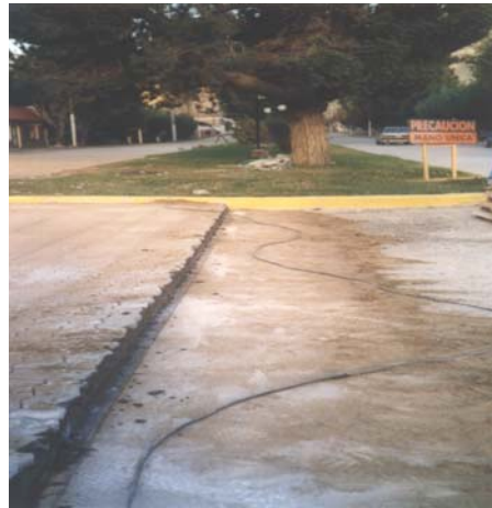
Figure 4. Metallic confining beam: steel angle fixed to the pavement.
