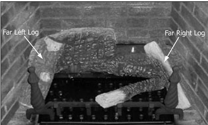
Figure 40. Third Stage Log Set Installation
