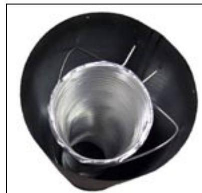
Figure 19: Wire Spacer in Place.
