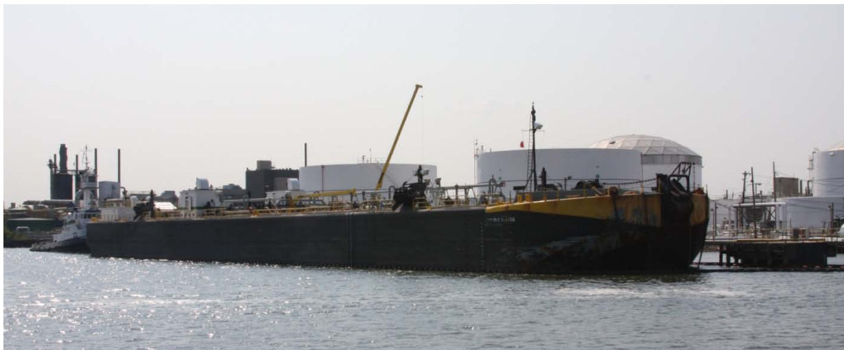
Figure 8. Sunoco Berth in the Kearny Point Reach, September 2008
