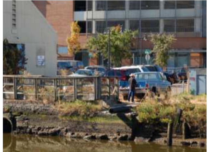
The Kiwanis Fishing Pier was demolished in anticipation of major improvements at the end of C Street. Photo: Nicholas Goulden
