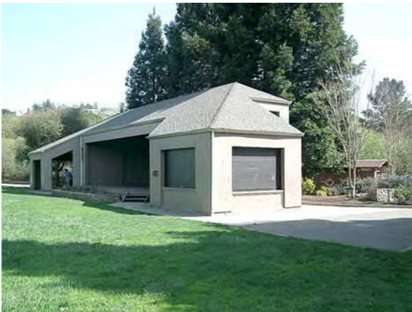
Northwest front corner of bandshell
