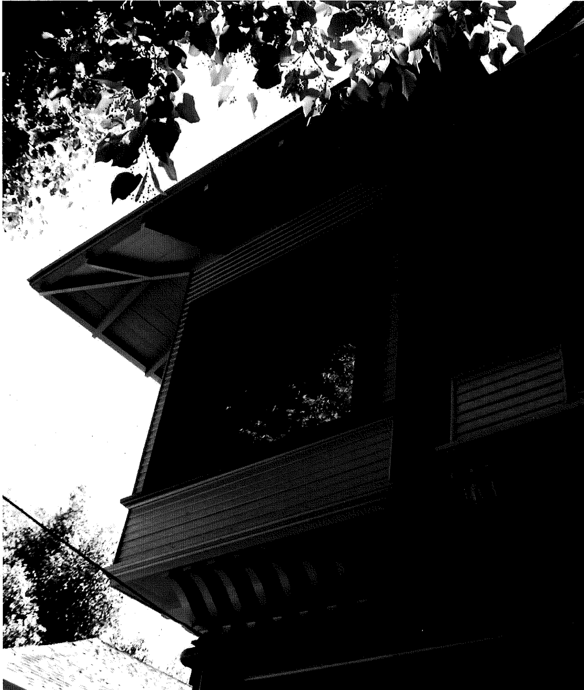
Detail view of second-story cantilevered corner bay window, viewed facing southwest.
