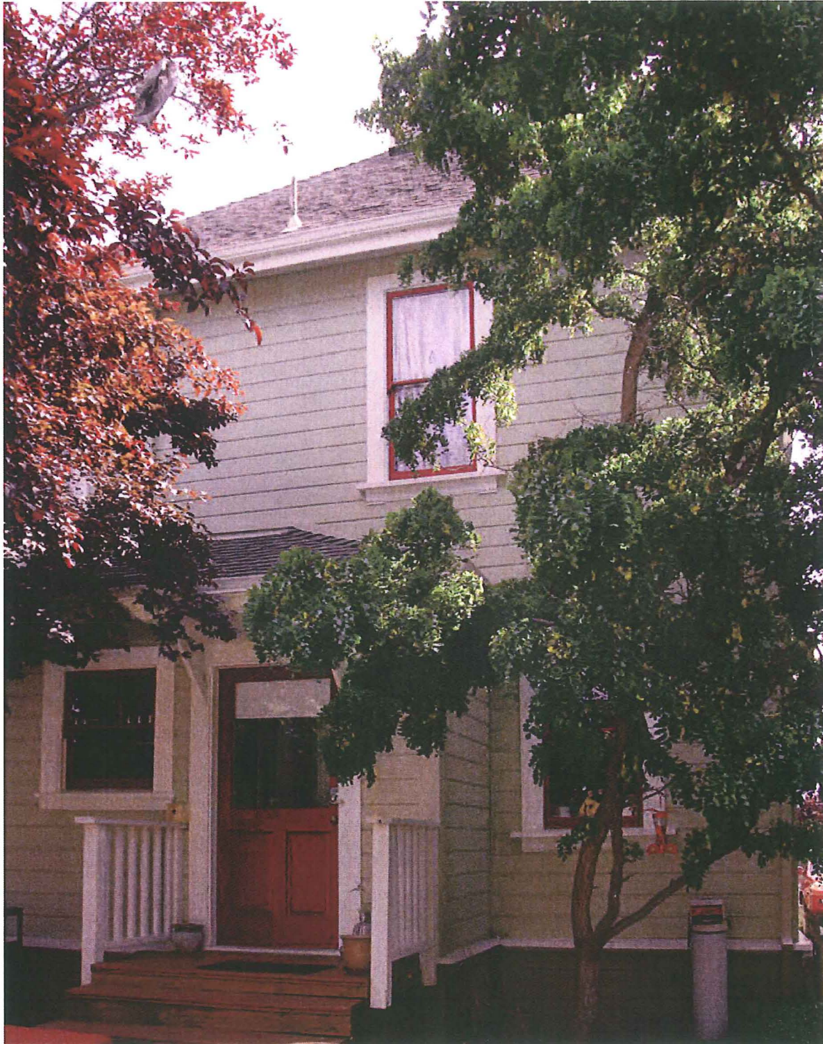
Rear elevation, viewed facing northeast.
