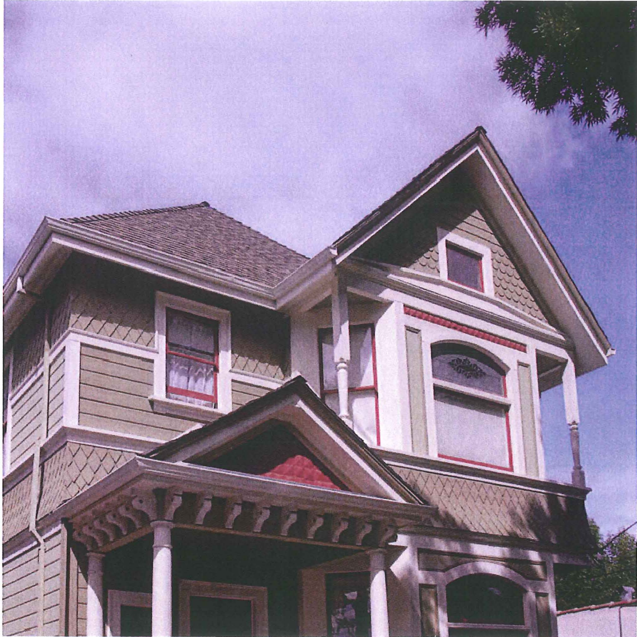
Detail view of front façade, viewed facing northwest.
