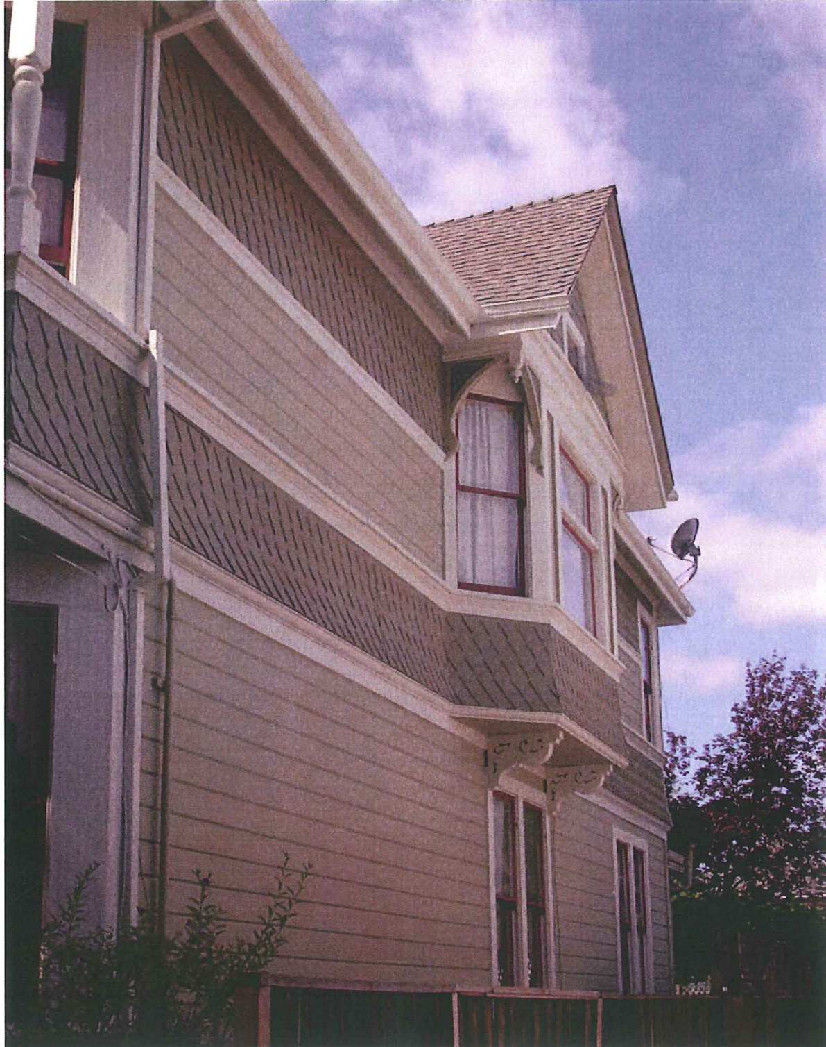
North elevation, viewed facing southwest.
