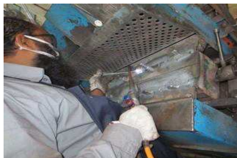
Figure 7.4: Group Burning with Lead Stick [2].
