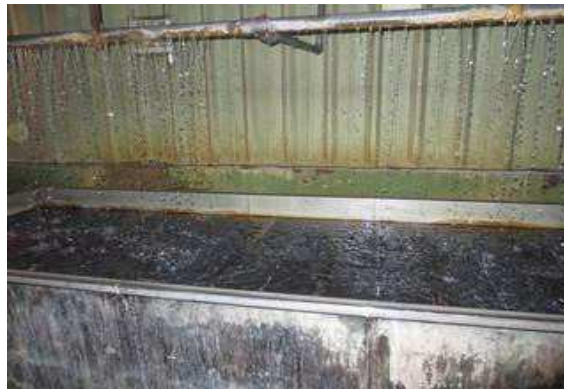
Figure 6.9: Washing Tank for Positive Plates [2].
