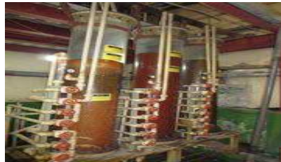
Figure 6.7: DM Water Plant [2].
