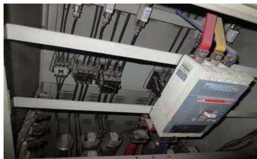
Figure 9.6: Capacitor Bank [2].
