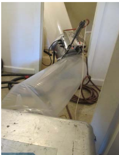
Aerosolized duct sealing helped reduce duct leakage to outside by up
