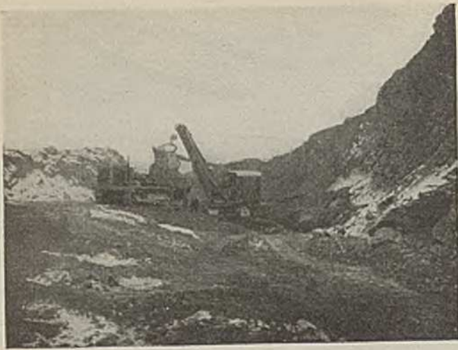
Fig. 3—Stripping the Orchard Bed, Kingston Colliery
