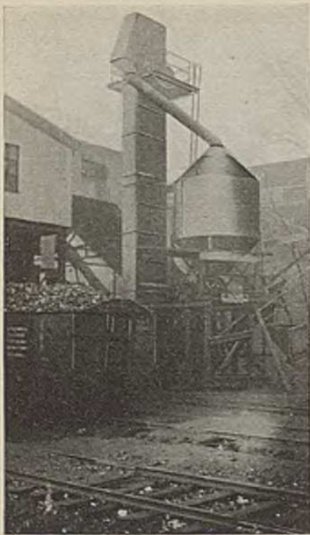
Elevator, Tank and Loading Terminal With Bucket in Position at Gate
