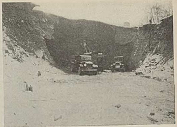
Fig. 4—Stripping Wash Over the Lance Vein, Kingston
