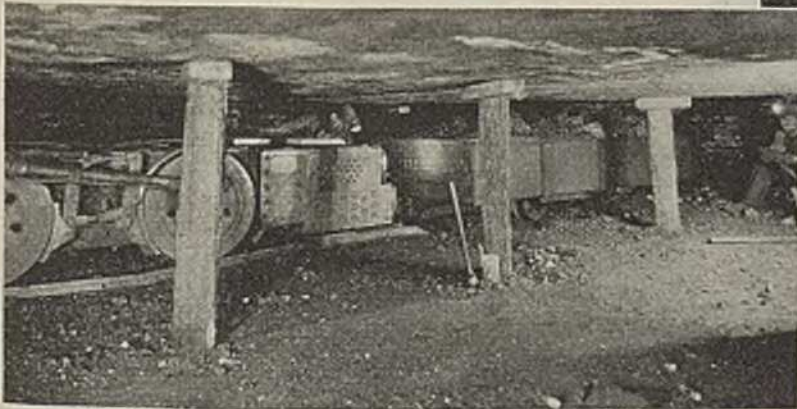
The Locomotive Has Arrived to Pull the Loaded Car From the Face and Replace It With an Empty.
