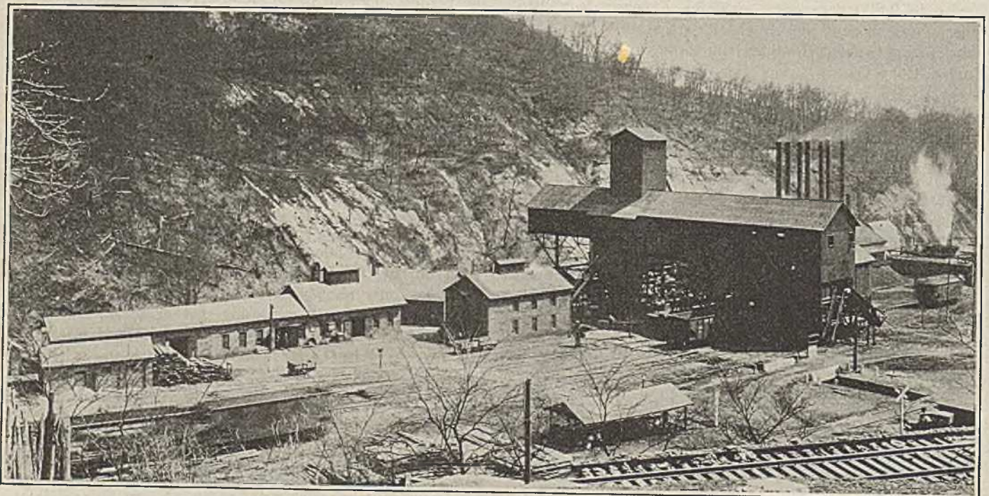
Fig. 2—Old Mine Plant now Practically All Gone
