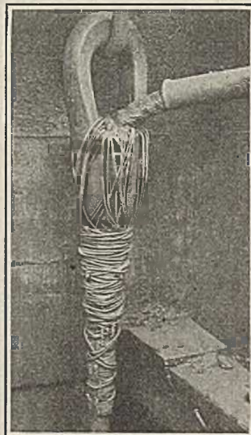
Close-Up of Cable Suspension
