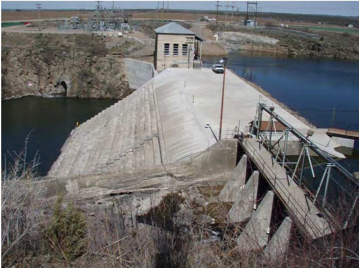
Figure 2.2-2 View of Ashton Dam showing spillway (foreground), powerhouse and substation (background)
