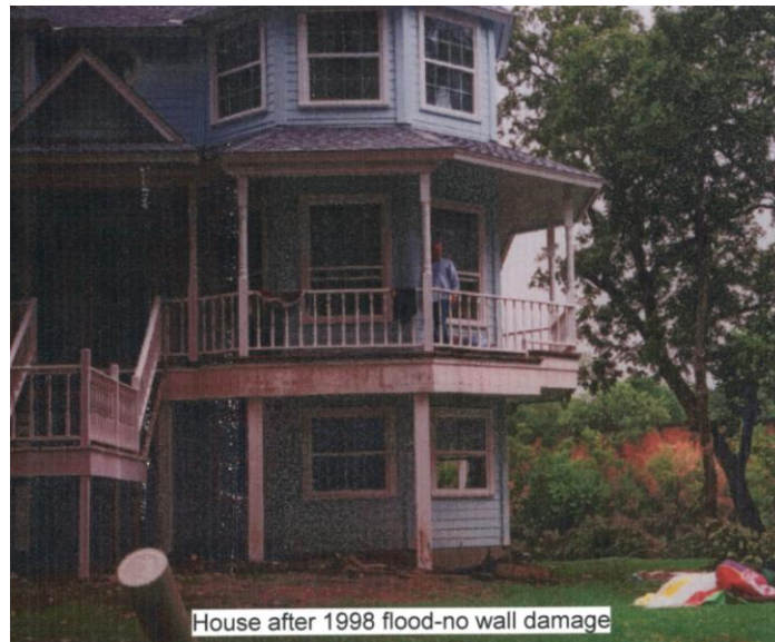
Figure 3 An ICF home withstands flood waters of Guadalupe River, Texas.
