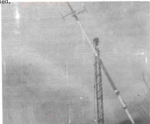
Crane lifts first mast at its' precise balance point.
