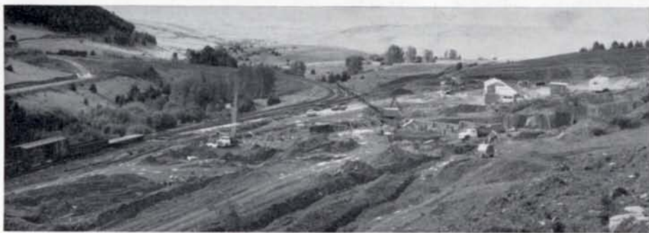
THIS PICTURE OVERLOOKS the site of the Douglas mill and the railroad yard tracks in the first stages of construction during July, 1963. In the background are a load track, a fill over Douglas creek and a view of the track leading down grade to Elephant.
