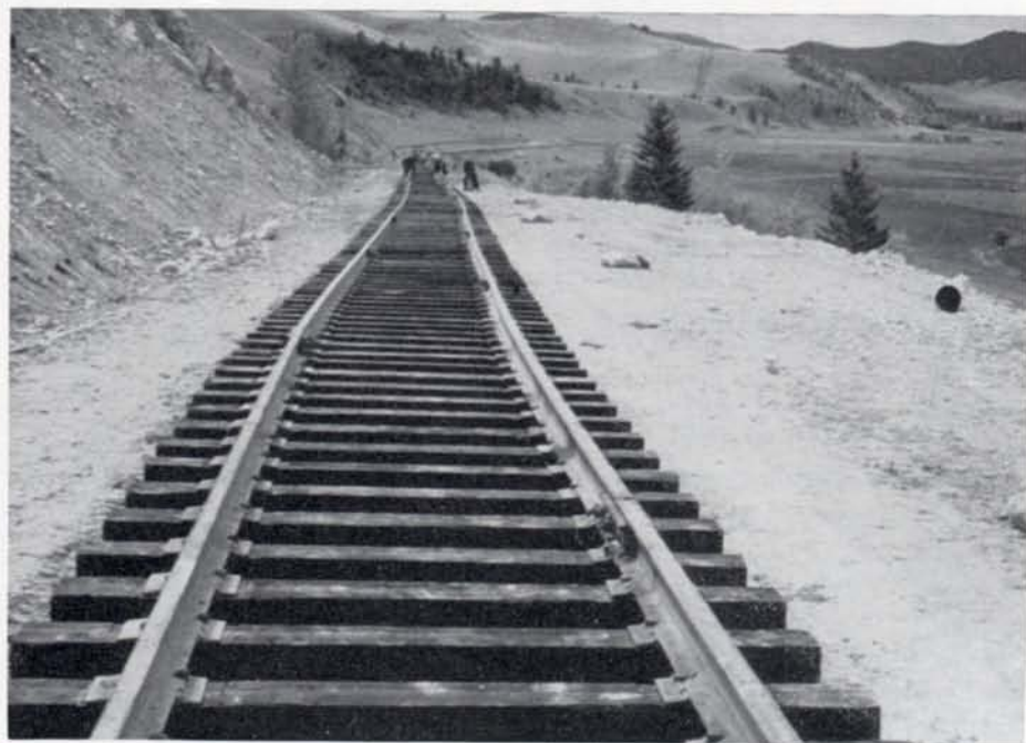
MEN LINE NEW TRACK near a two per cent ascending grade on a spur built last summer to the Douglas concentrator of the Montana Phosphate Products company. The track required considerable lining prior to ballasting on account of the grade.
