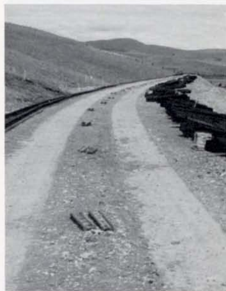
TIES AND 131-POUND RAIL WERE distributed along the grade of new spur for a mining and milling project with trucks and then were assembled in nearly record time with Quickway and Speed-Swing cranes and a section crew with 24 men.
